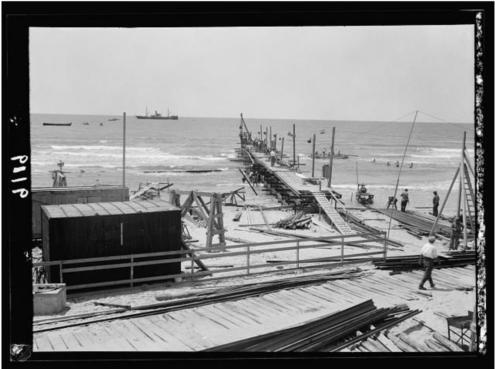
Construction of the
